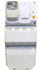
Directly coupled to a Lucy heavy duty cut out.
