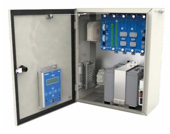
Designed for advanced feeder automation in electrical distribution networks.
