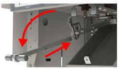
**5** : Once star point earth bar is clear from all the bushings, remove the operating handle. Test connections can be now made onto the bushings.
