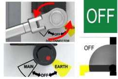
5 : Remove' CIRCUIT BREAKER' padlock if fitted and pull down the slide cover to the 'unlocked' position.With the operating handle on the 'CIRCUIT BREAKER' boss, rotate the ratchet mechanism 360° clockwise. The ratchet mechanism enables this operation to be carried out in multiple small rotations. At the end of the operation the 'CIRCUIT BREAKER' will close to main 'EARTH-ON'.
