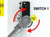
3 : Rotate the 'SELECTOR' knob anti-clockwise to 'MAIN SWITCH'.
