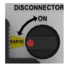
4: With the operating handle on the 'DISCONNECTOR' boss, rotate anti-clockwise into 'EARTH-SELECTED'.
