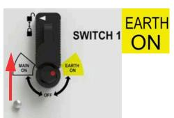
5: With the operating handle on the switch boss, rotate clockwise until the switch opens '**OFF**'.
