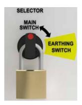
Lock the 'CABLE TEST ACCESS SELECTOR' using the padlock, as show below.
