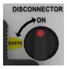
6: With the operating handle on the **DISCONNECTOR** boss, rotate clockwise into 'MAIN'.
