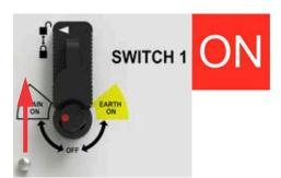
2: With the operating handle on the switch boss, rotate anti-clockwise until the switch opens 'OFF'.
