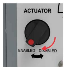
Rotate the selector to '**DISABLED**' for manual operation of the load break switches.
