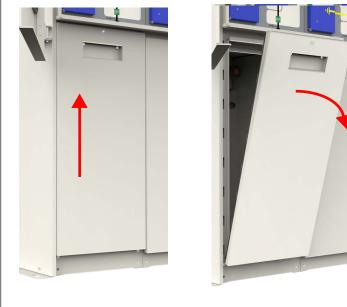
NOTE: The relevant function cannot be removed from 'EARTH-SELECTED' until the cable box cover is refitted.
