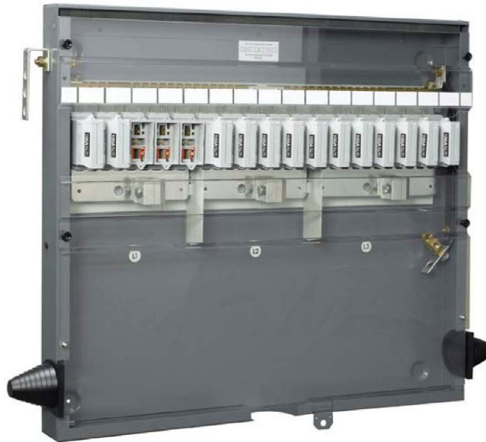
16-way Version Shown With Cover Removed
