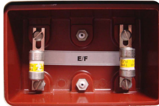
Fuse dimensions: Length 57mm x Diameter 13mm
