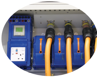
Standby generator cables fitted to the Veam Powerlock sockets. The earth socket is mounted at the bottom of cabinet.
