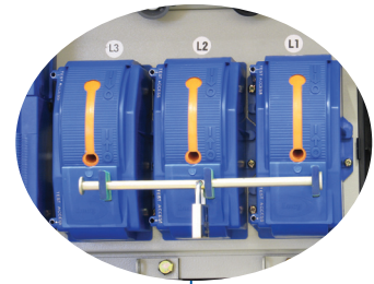
Transformer disconnectors padlocked off with the link bars in place.
