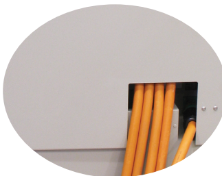
Aperture in lower edge of door allows five generator cables to exit the cabinet with the door padlocked shut.
