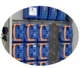
Transparent fuse way shield padlocked in place.
