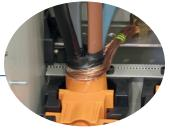
Cleats are load bearing and provide a solid anchor point during cable connection.
